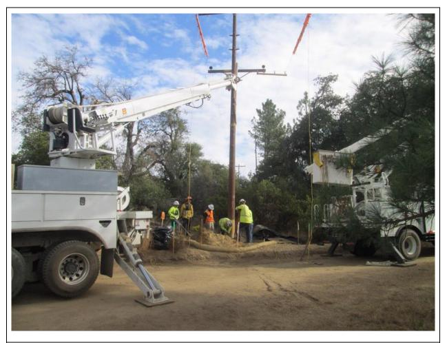
**Photo 1**: A construction crew observed setting a direct bury steel pole (C 442). Fiber rolls were present and functional in accordance with the project's Erosion Control Plan, SWPPP (MM HYD-1, MM BIO-7) and APM HYD-09.
