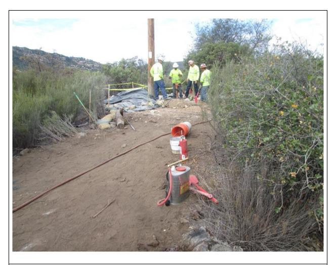
**Photo 2:** A construction crew observed trenching and installing ground rods at Pole P177017 (C442). The crew was observed staging the required 5-gallon backpack pump, round point shovel, Pulaski, and 2A10BC fire extinguisher, along with 100 gallons of water and pump hose (not pictured) in accordance with the Fire Prevention Matrix (off CNF land), CFPPP (MM FF-1 and APM HAZ-01), and APM HAZ-04.
